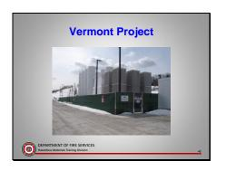
A Large Gypsum producer in central Vermont is currently in the process of installing eight 15,000 gallon fixed LNG storage tanks to replace their use of #2 Fuel oil.
