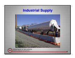
The northeast is now beginning to see the use of LNG as an alternative to Propane. LNG storage tanks are connected to portable/fixed vaporizers and odorant stations. This system in NH is being used to replace a 30,000 gallon LP tank. (Shown back left at base of smokestack)
