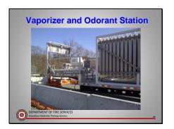
Dual vaporizers alternate on a 12 hour cycle due to icing. Methane vapors are odorized with Mercaptan and the gas is heated to 40 degrees Fahrenheit before entering the facility.
